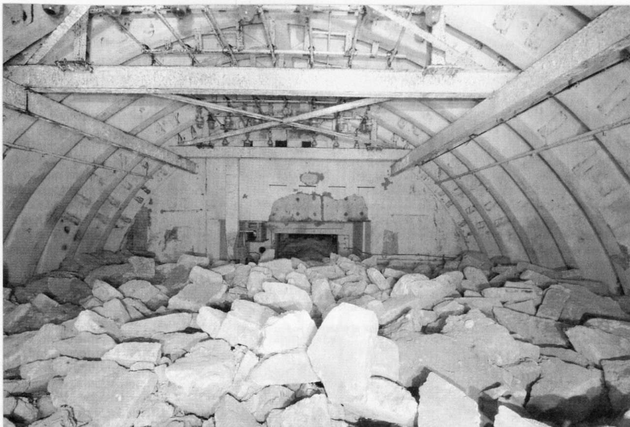
The nuclear warhead store adjacent to the Soviet airbase at Nobitz - Photo Dan McKenzie
